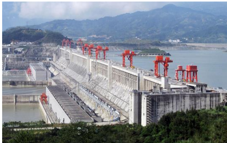
Fig.2. hydro power plant
