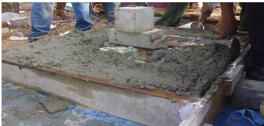
**Fig 4.4 Concreting of Infill Wall Panel**
