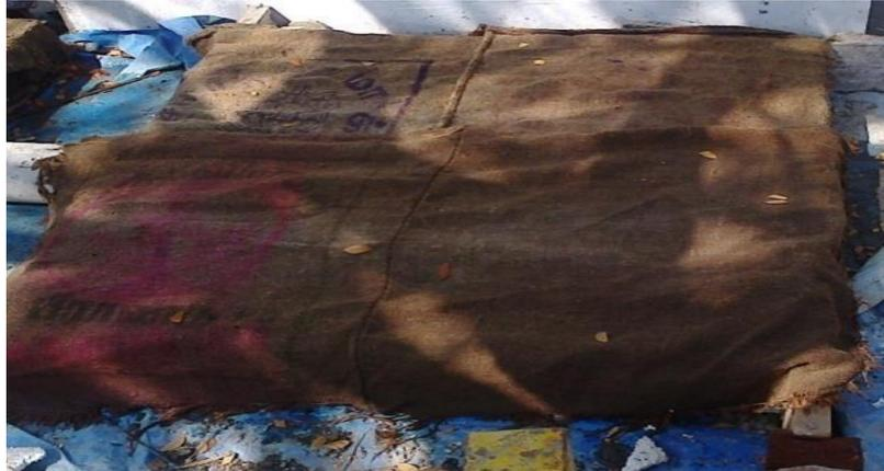
**Fig 4.5 Curing of Infill Wall Panel**
