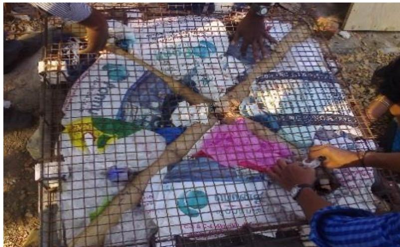
**Fig 4.2 Bamboo as Diagonal Struts and Waste Plastic Bags as Infill SBA-2**
