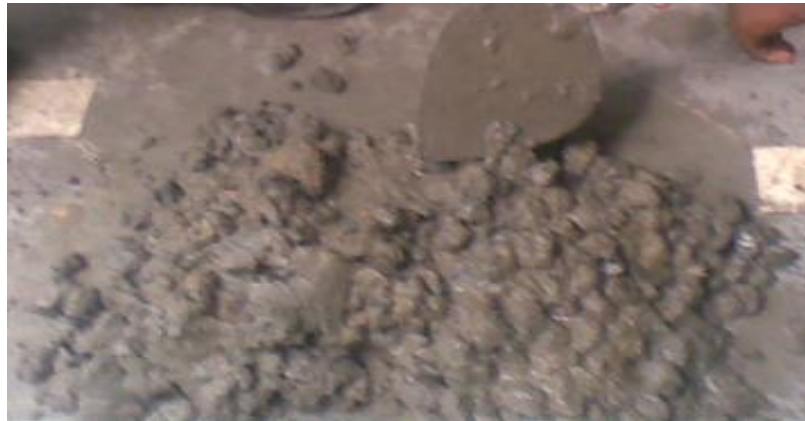
Fig 3 -Mixing of concrete
