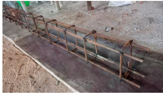
Fig Beam reinforcement
