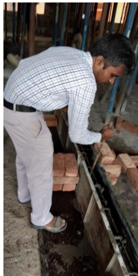
Fig Beam casting
